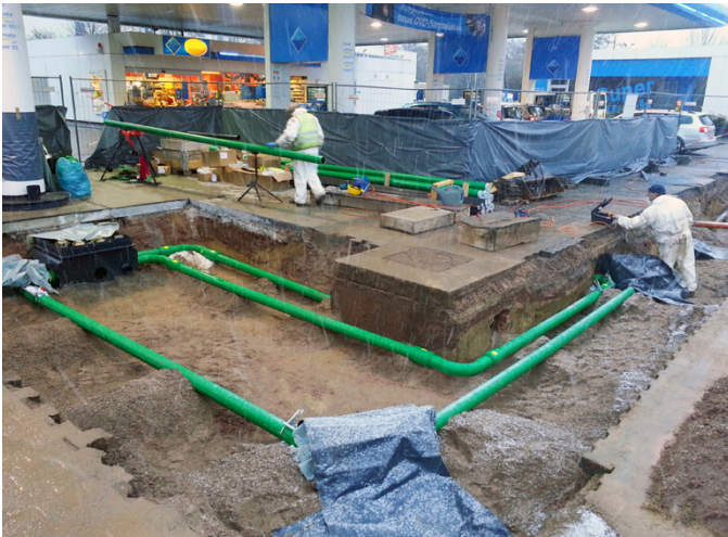
KPS' quick and easy installation resulted in no interruption of fuel sales
