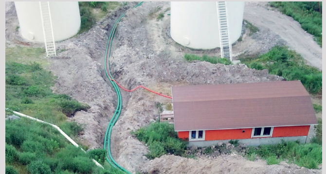
EDF Termik Santrali, Saint Pierre, Fransa
