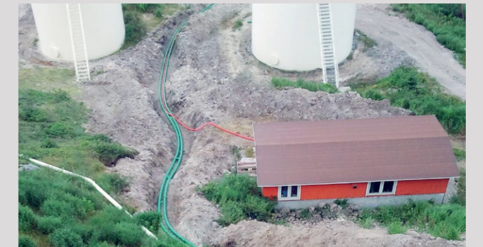
EDF Termik Santrali, Saint Pierre, Fransa
