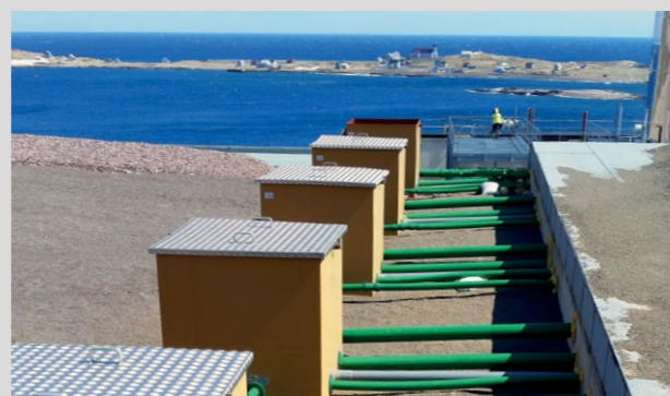
Thermal Power Plant, France
