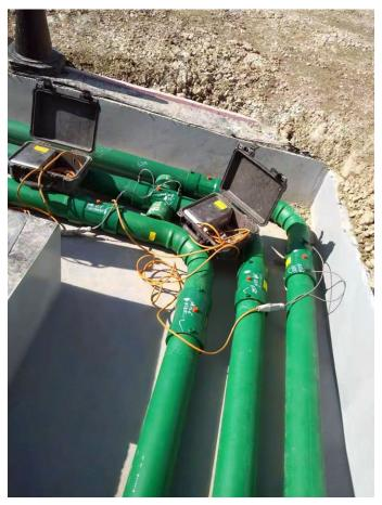
KPS electrofusion welding, ensures the piping system has zero permeation (liquid/watertight).
