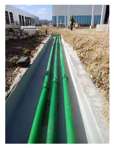
KPS' double wall piping includes an interstitial space, providing an extra layer of security.
