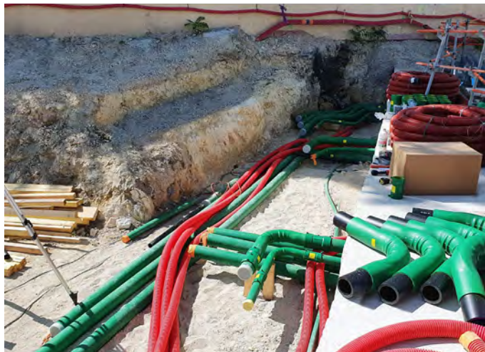
KPS' double wall pipework includes an interstitial space between the inner and outer pipes, providing an extra layer of security
