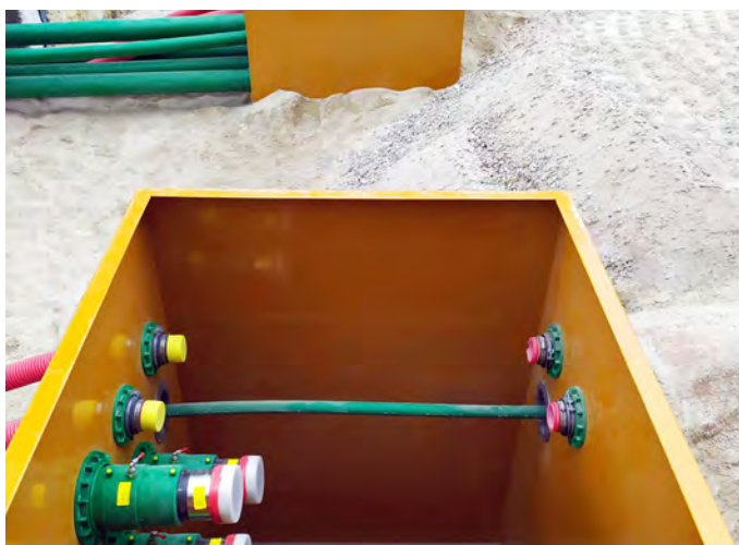
KPS 4" piping allows a flow rate of 933 litre/minute enabling fast fuel delivery
