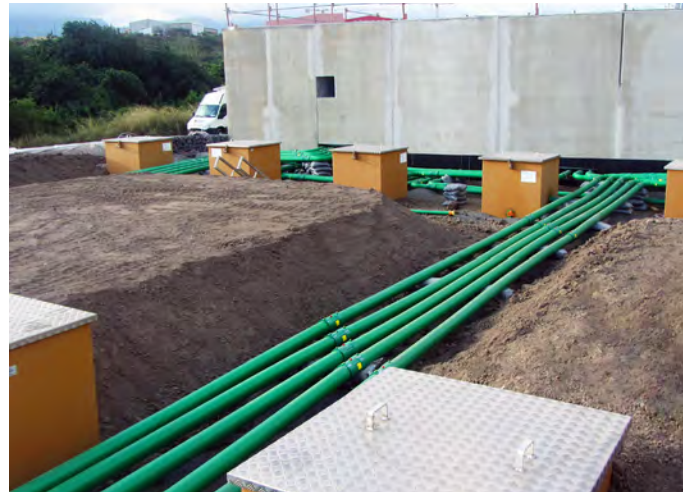
KPS' conductive piping is electrostatically safe, avoiding potential static build-up
