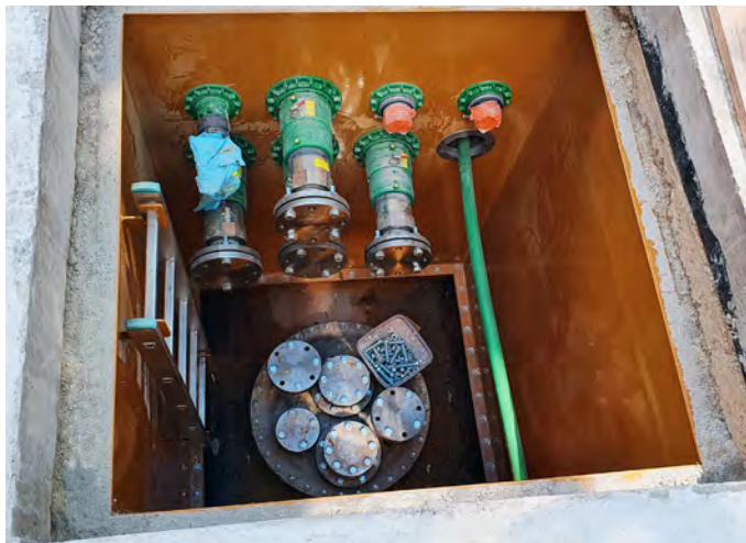
KPS provided a liquid tight solution, including watertight entry boots
