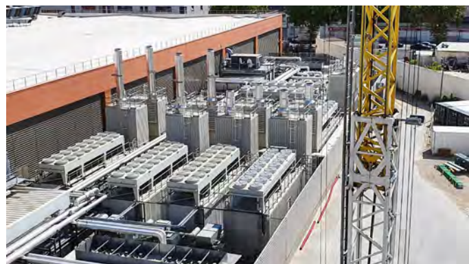
Data centre facilities require a number of backup generators to ensure an uninterrupted power supply
