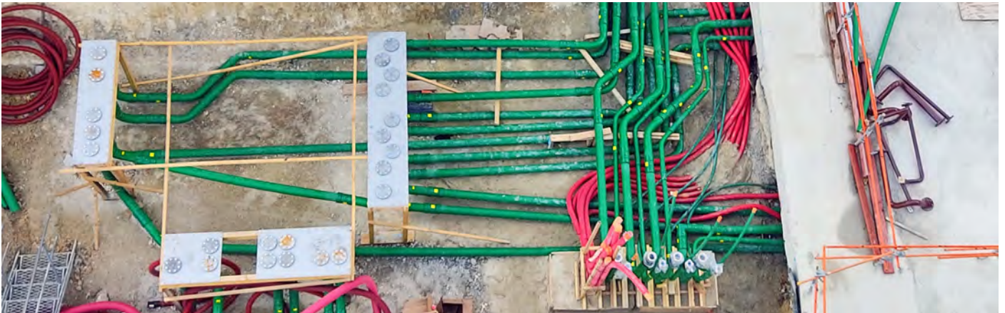
A new data centre facility in Paris, France specified KPS double wall piping to fuel backup generator
