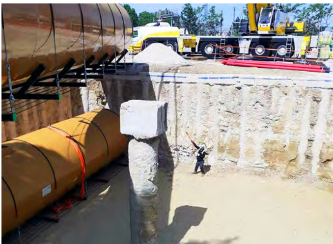
KPS conductive 4" pipe (125/110mm) was installed to connect the remote filling point to the fuel tanks
