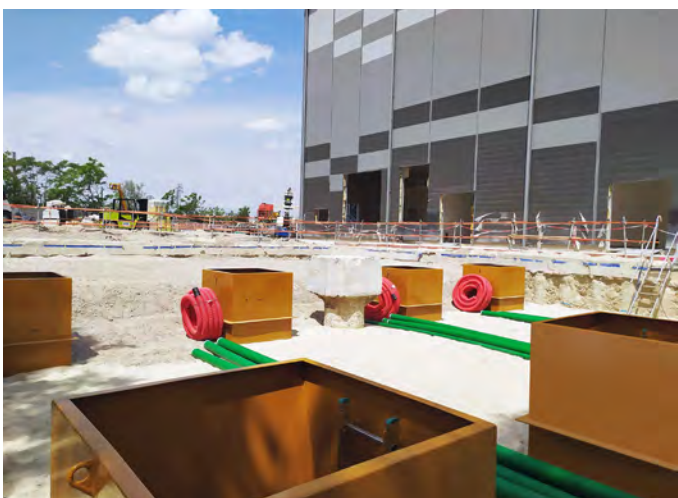
KPS 2" (75/63mm) conductive double wall piping connects fuel tanks to backup generators
