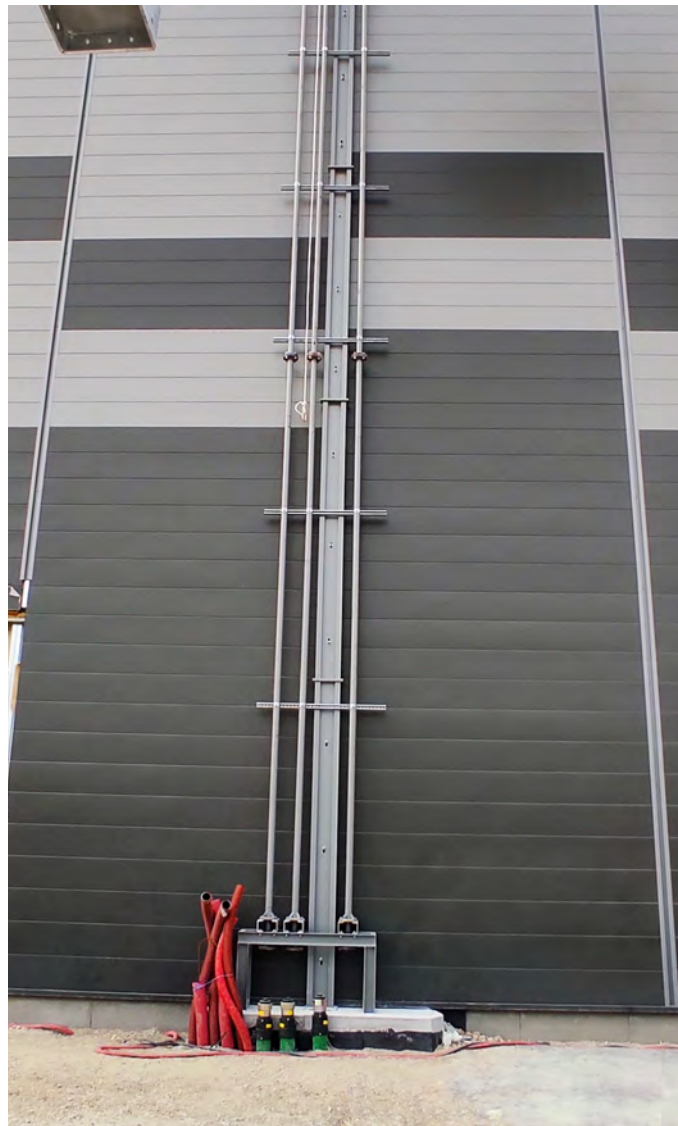
KPS' 2" (75/63mm) double wall piping was installed to connect fuel tanks to metal piping running up the outside wall of the facility
