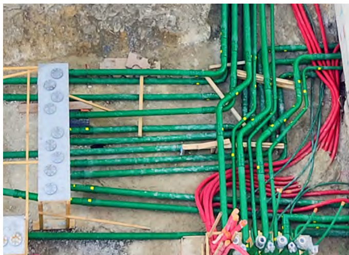
Conductive KPS piping is electrostatically safe, preventing potential static build-up
