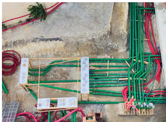
KPS' 4" (125/110mm) double wall piping was installed to connect remote fill points and below ground fuel tanks
