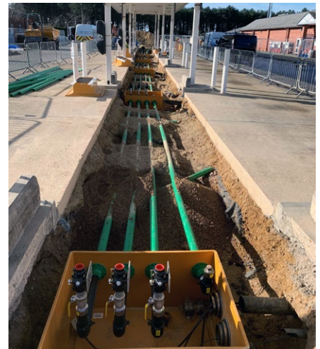
Custom 10m lengths of KPS straight pipe simplified installation
