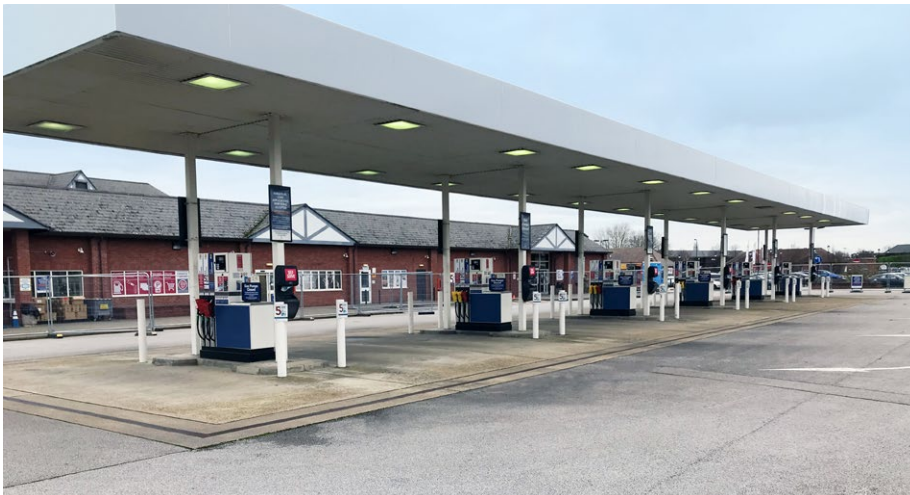
KPS & Fibrelite provided a retrofit liquid-tight solution at this UK military refuelling facility
