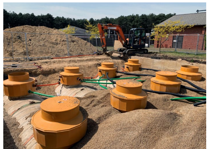
KPS double wall piping and Fibrelite tank sumps ensure complete containment and conductivity
