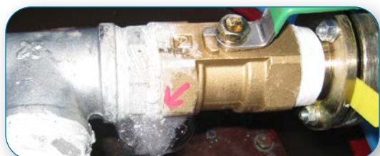
The formation of bubbles is a sure indication of leakage.
