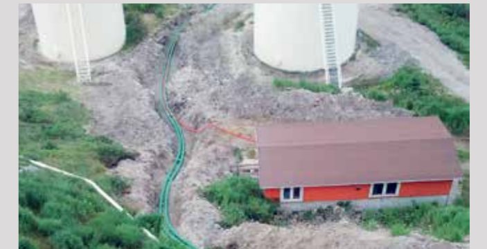
EDF Termik Santrali, Saint Pierre, Fransa
