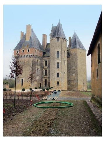
KPS installed a remote filling point 60 metres from the Château, connected to the diesel fuel tank with KPS conductive double wall piping.
