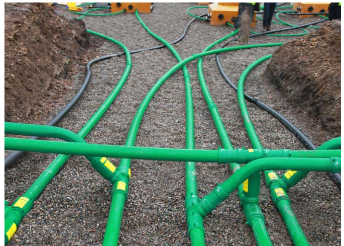
All integrated double wall KPS fittings weld both pipe walls simultaneously.
