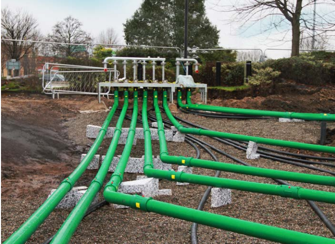
KPS formed bends below fill point.
