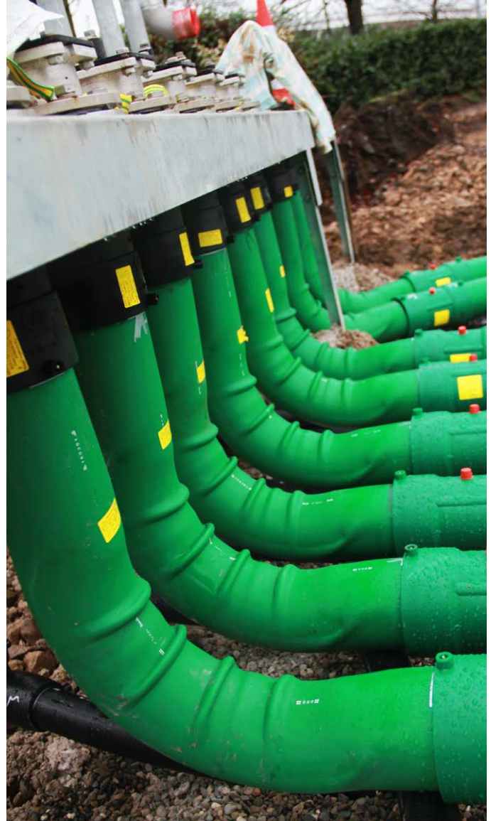
KPS bends below fill point.
