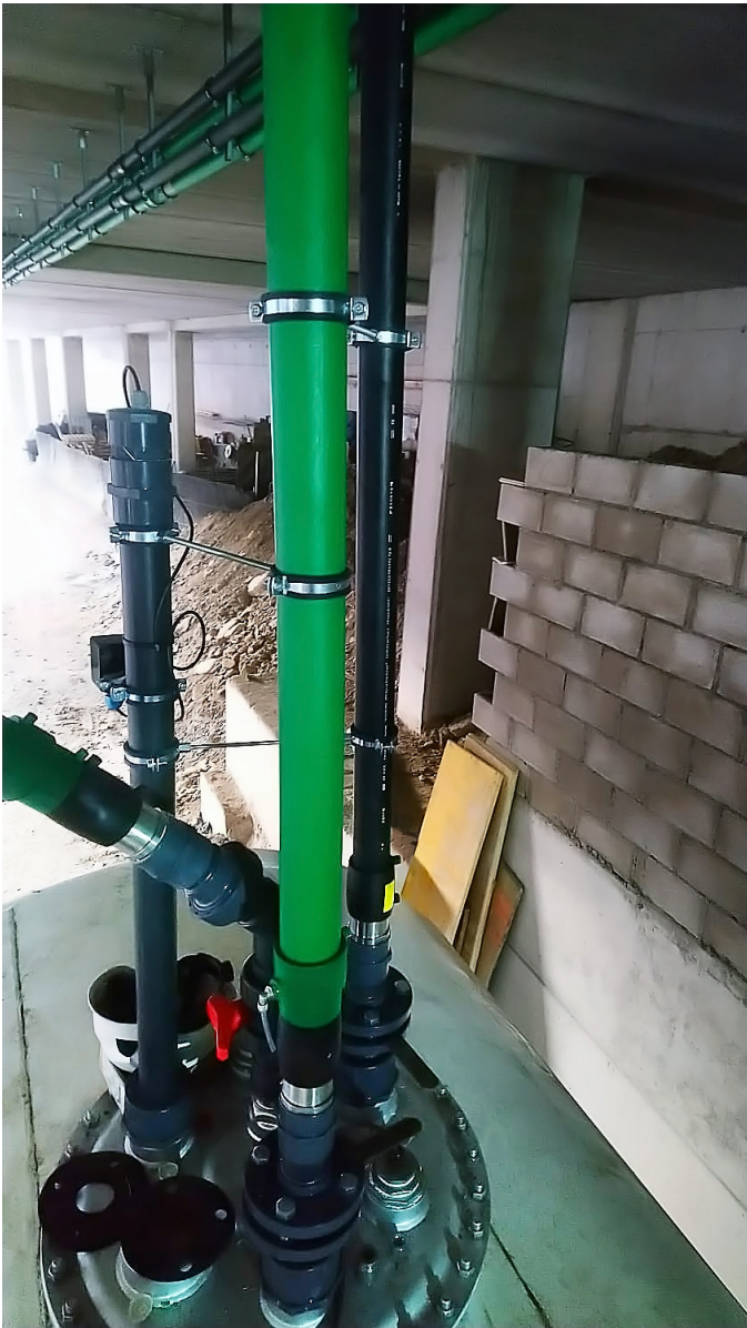
KP 75/63 double wall and KP 63 single wall piping connected to the above-ground tank. A leak detector is also connected to the interstitial space of the double wall pipe
