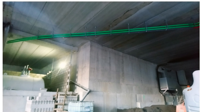
KPS 75/63 coiled pipe is optimal for long pipe runs, negating the requirement for additional/unnecessary welding sockets
