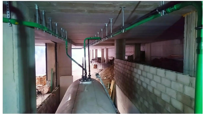
Above-ground diesel tank: KPS piping was installed on the roof of the gallery using metal supports
