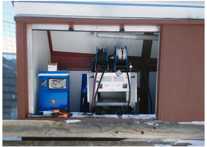
KPS piping connects the above-ground tank to the outdoor refuelling area.
