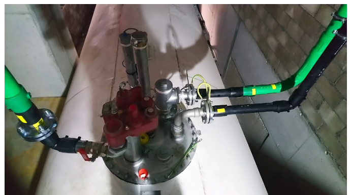
KPS' conductive piping can easily be earthed to prevent electrostatic discharges. The yellow cables required for this are connected at the end of the pipe run
