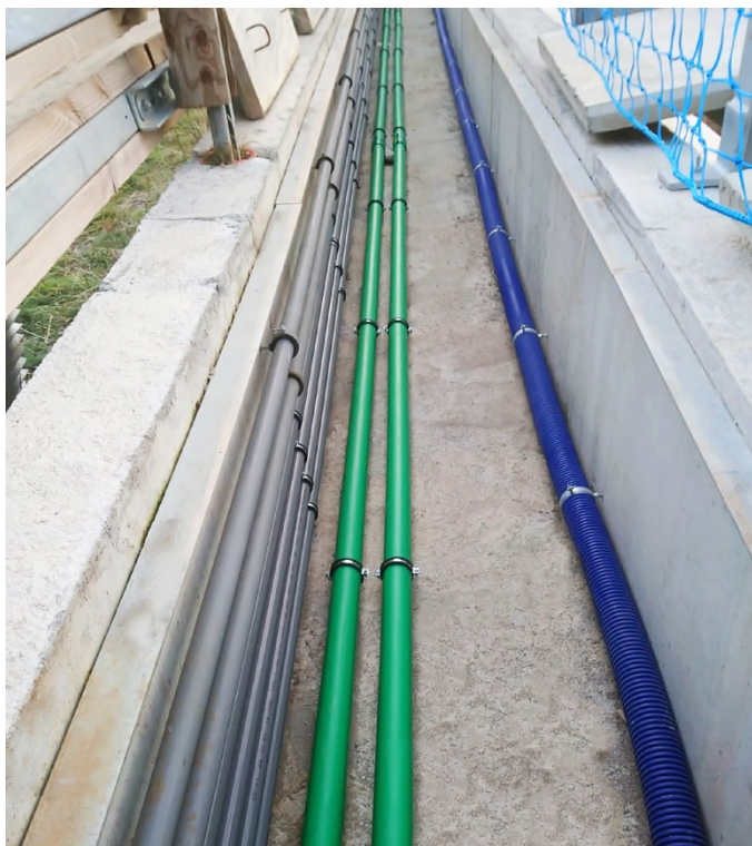
KP 75/63 double wall pipe coils were installed in a concrete trench around the ski resort
