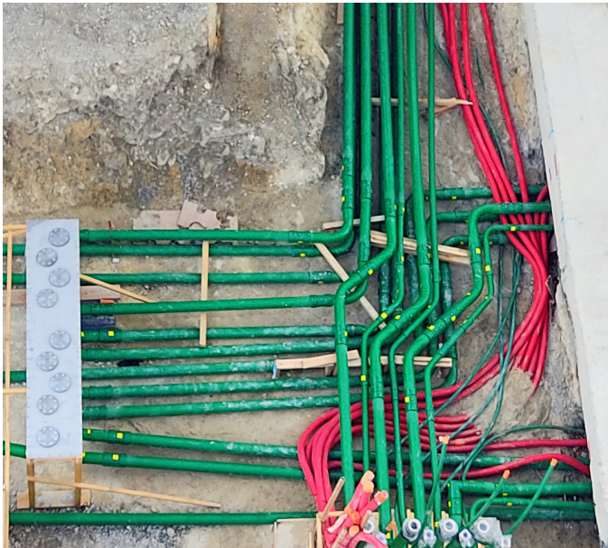
Conductive KPS piping is electrostatically safe, preventing potential static build-up
