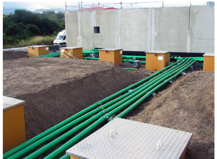
KPS' conductive piping is electrostatically safe, avoiding potential static build-up
