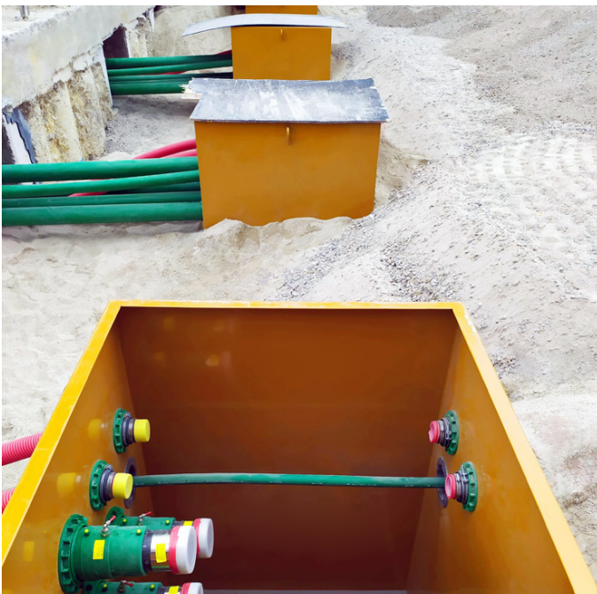
KPS 4" piping allows a flow rate of 933 litre/minute enabling fast fuel delivery
