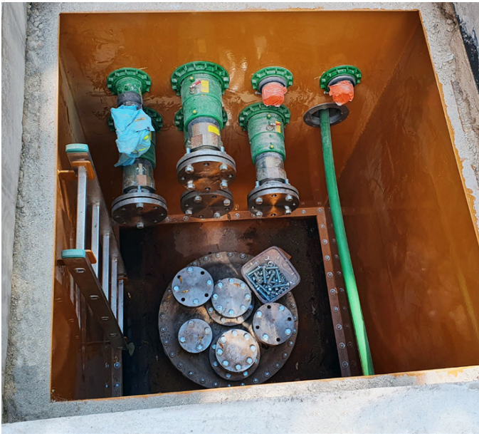
KPS provided a liquid tight solution, including watertight entry boots
