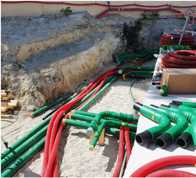
KPS' double wall pipework includes an interstitial space between the inner and outer pipes, providing an extra layer of security
