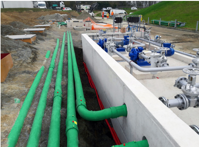
KPS conductive double wall piping provides the highest possible level of safety for Ethanol's potential to generate charge
