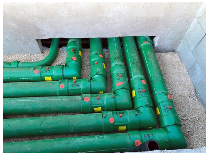
KPS 4" double wall 90° pipe elbows are a compact solution for projects where space is tight
