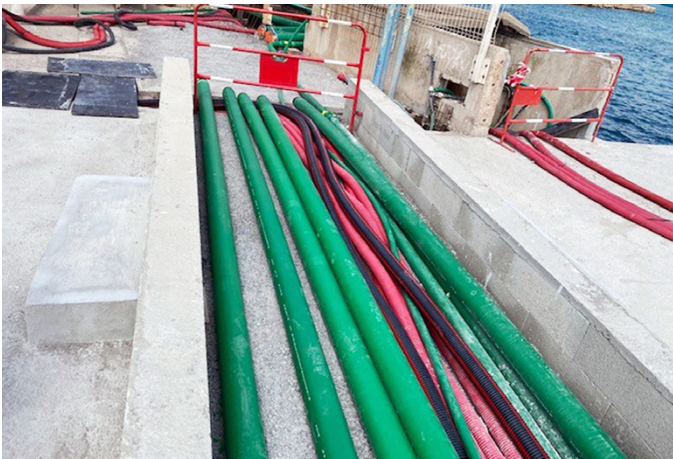
KPS piping includes an EVOH permeation barrier and a conductive layer of carbon black
