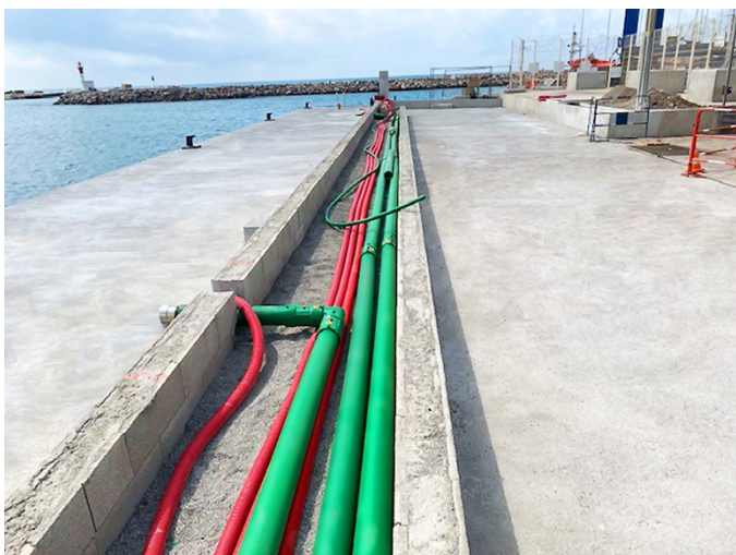
KPS 4" double wall pipe (125/110mm) provides a 933 litre/min flow rate
