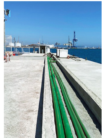
KPS 4" piping allows a flow rate of 933 litres/minute enabling fast fuel delivery
