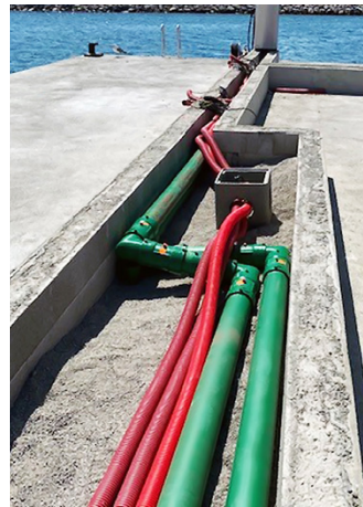
Conductive KPS piping is electrostatically safe, preventing potential static build-up
