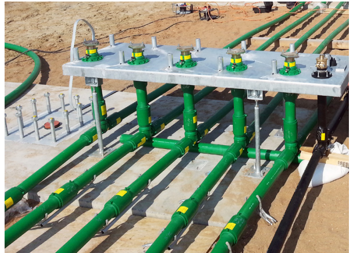
KPS provided an installer friendly solution to meet BP-Aral's strict project deadline
