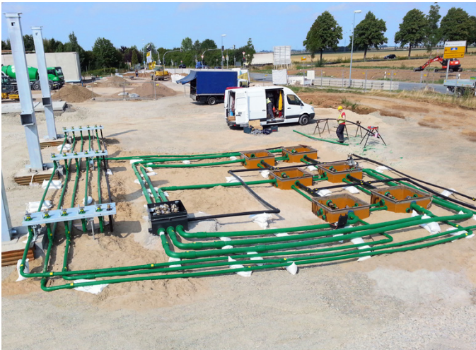
BP-Aral specified KPS' plastic double wall piping at a new build site in Hildesheim, Germany
