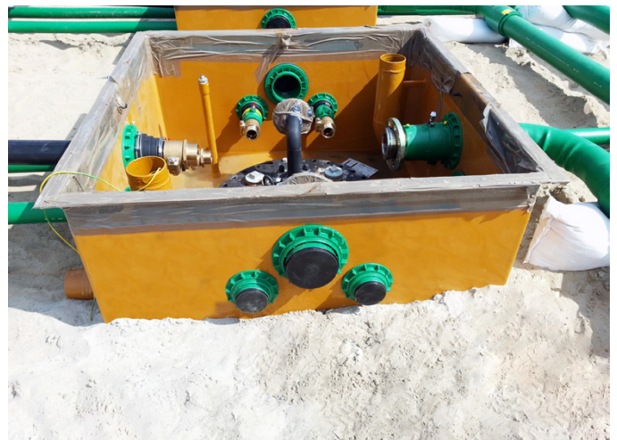
Tank chambers were supplied with pre-made holes on all chamber walls
