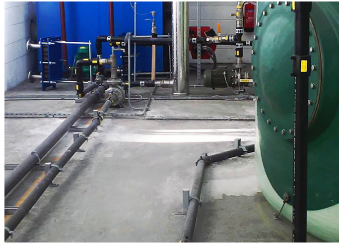
KPS piping is made of high-density polyethylene, and includes liners to prevent permeation of fuel
