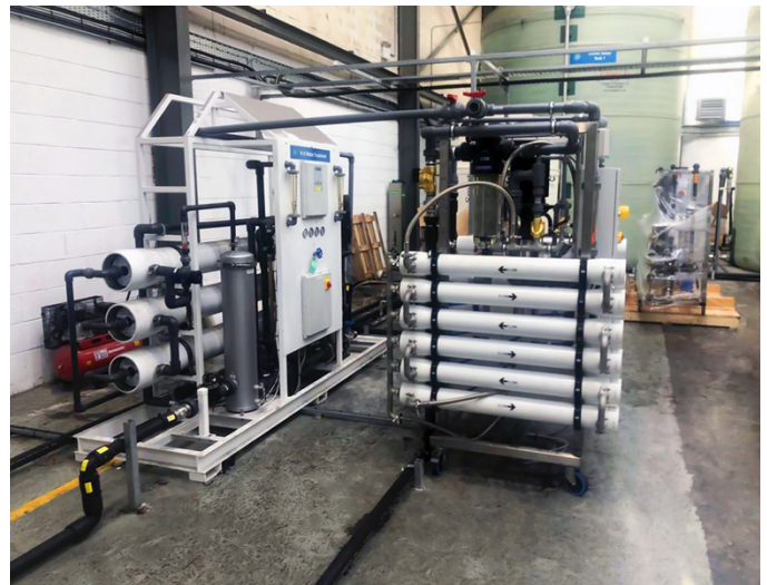
The installation was completed ahead of schedule
