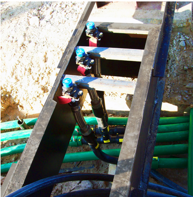
Sinooil required a solution that allowed emergency valves to be installed under dispensers
