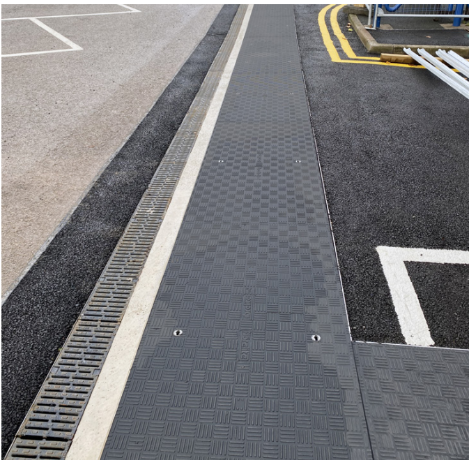
Fibrelite covers are corrosion-resistant, unaffected by water, underground gasses and most chemicals
