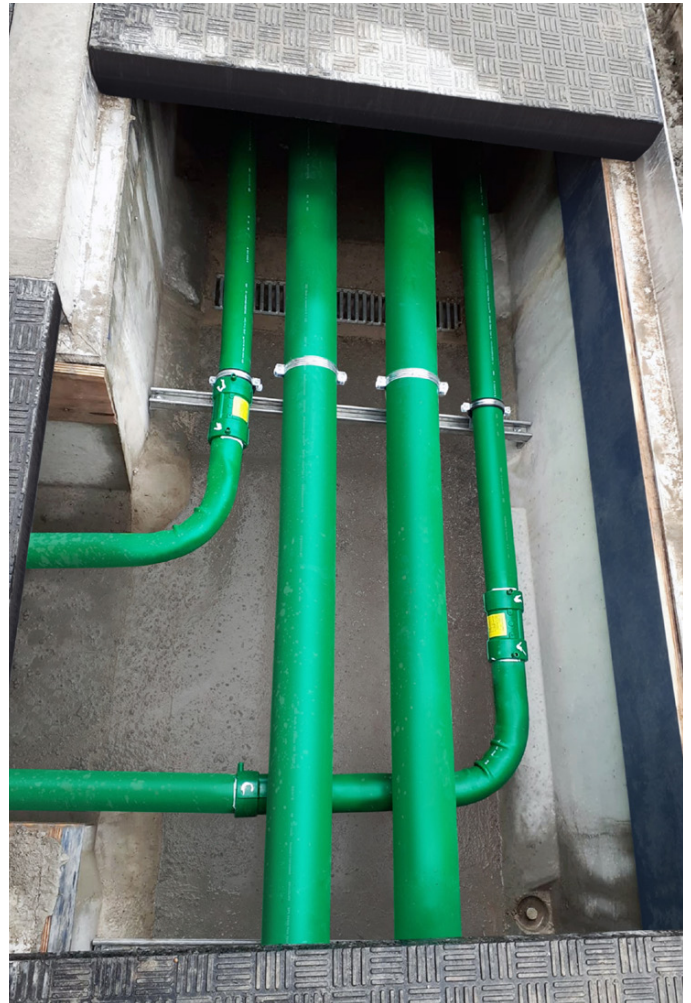
Quick access to piping is vital for maintenance and inspection
