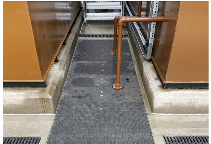
All trench covers can be safely removed manually by two people while strong enough to withstand sustained loading
