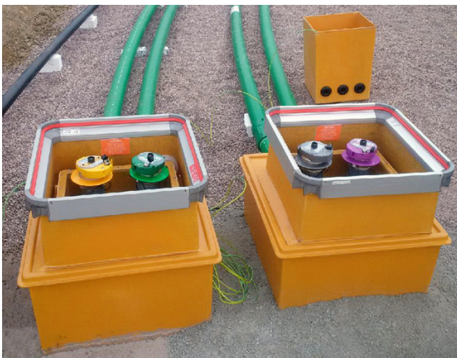
Below ground remote fill systems incorporating a sump and offset corbel with alternate pipe exit positions
