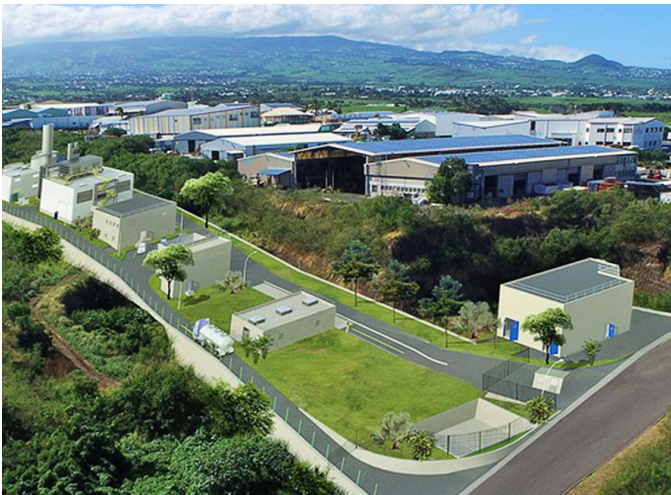
Multiple contractors were working at once on the Reunion Island site
